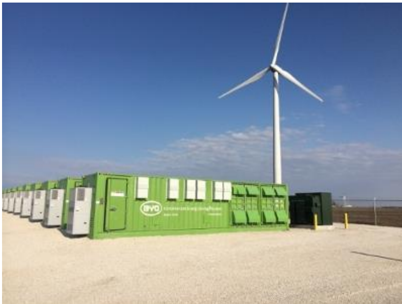
Figure 1-16: Invenergy Facility in Grand Ridge, Illinois
